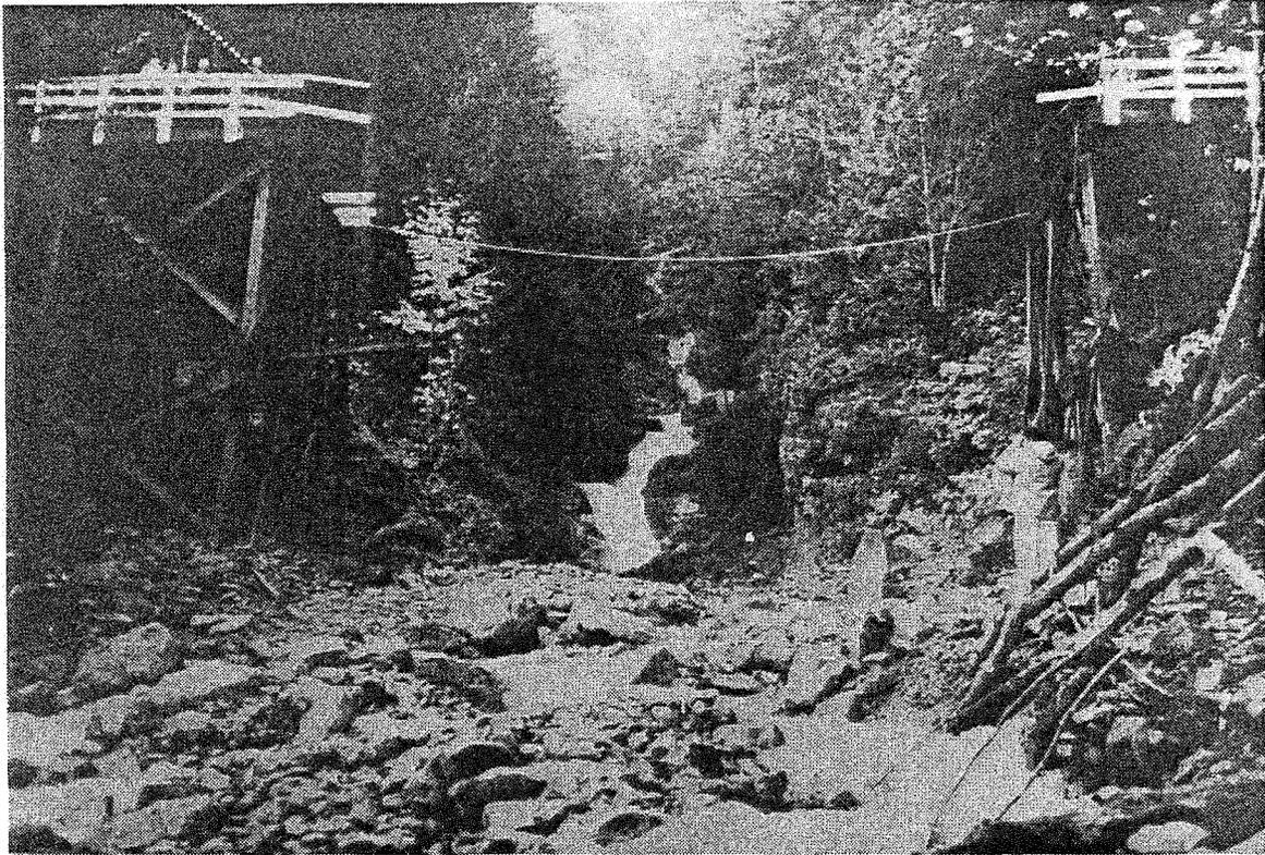
Figure 4 Highway bridge over M-Creek, shortly after its destruction by the October, 1981 debris flow.
